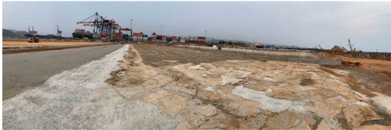
Construction of Main yard. (VCT-2)
