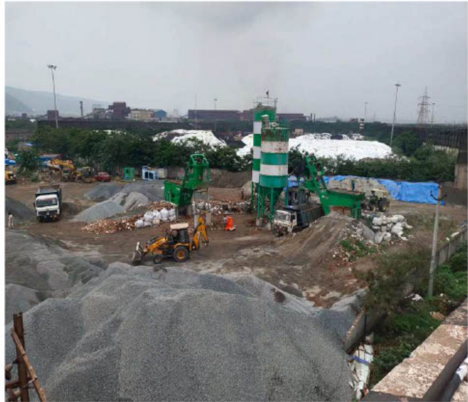
Batching Plant for Production of DLC for Yard formation. (VCT-2)
