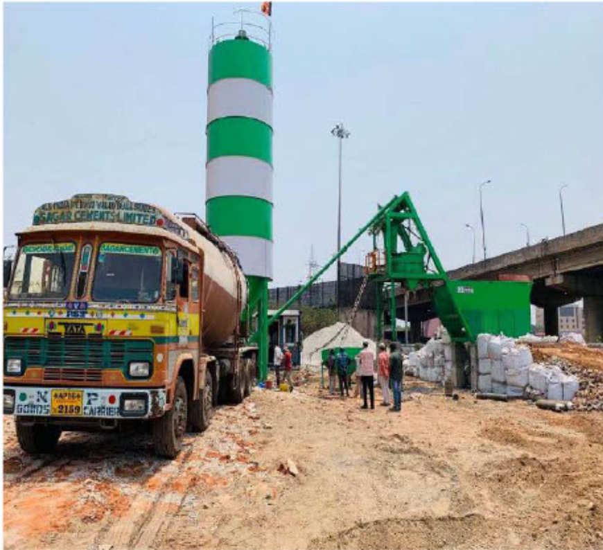
Batching Plant for Production of DLC for Yard formation. (VCT-2)
